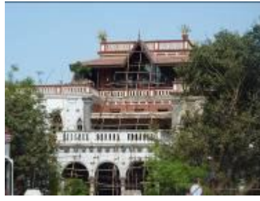
Mangaldas Heritage Boutique Hotel, Ahmedabad, India (Photo: Adishakti, 2012)
