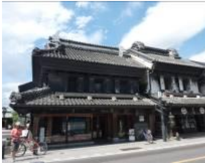
The Kura-tsumuri buildings
